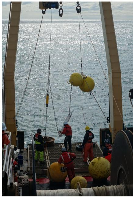
Figure 1. Mooring deployment in 'N' shape.
